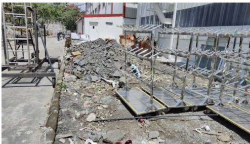
Landscaping work under progress
