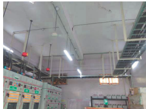
Internal view of Utility Building
