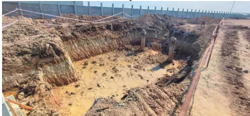
View of Bin Cleaning Shed & Meter Room
