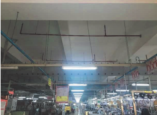
Internal view of Main Shed Ground Floor
