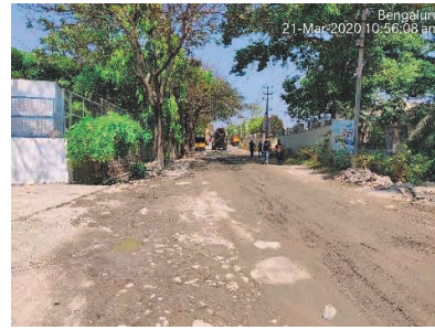
View of access road
