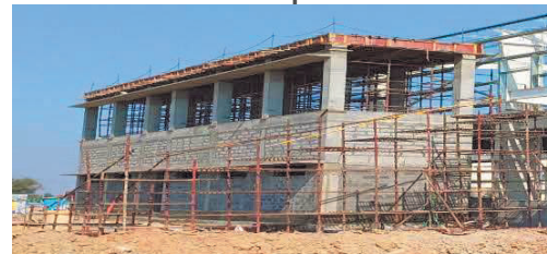
View of Rest Rooms
