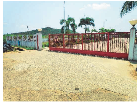
View of Entrance of the property
