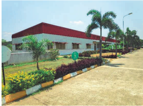
View of the canteen cum kitchen
