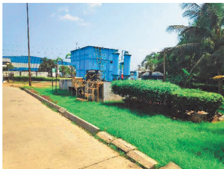
View of the Pumphouse
