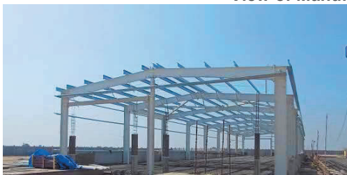
View of Utility Building
