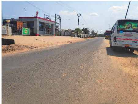
View of access road
