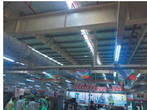
Internal view of Main Shed First Floor
