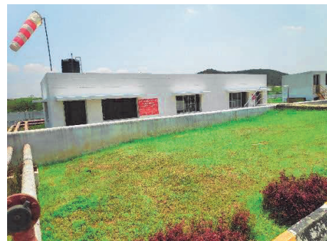
View of the pump room
