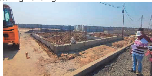
View of Kitchen Shed
