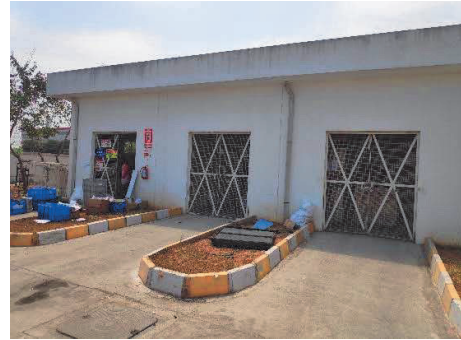
View of the diesel storage & scrap yard
