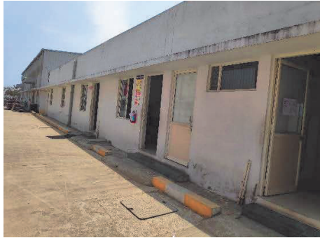
View of the ambulance room & creche
