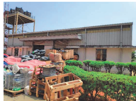
View of the wire storage room
