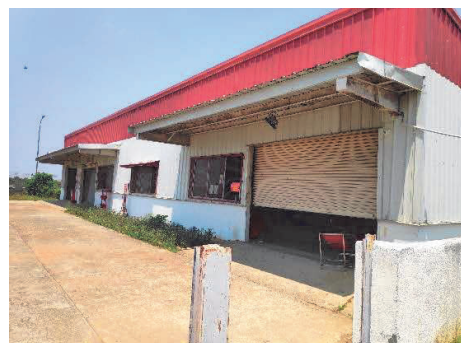
View of the utility Room
