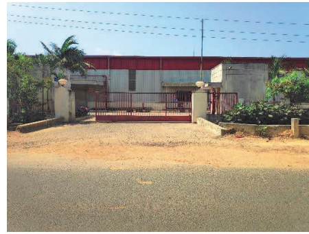
View of Entrance of the property
