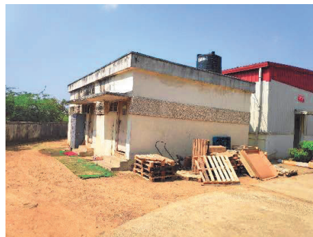
View of the rest room block
