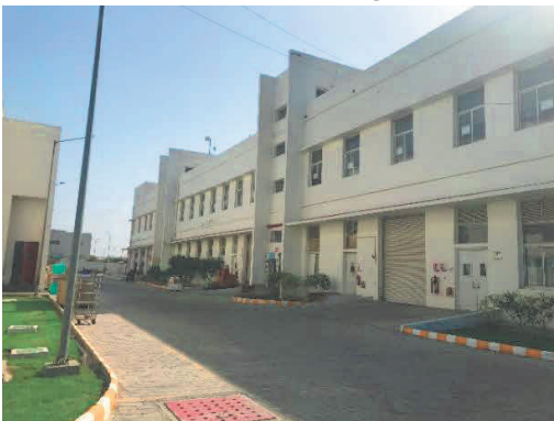
External view of Utility Building
