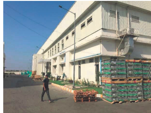
External view of Main Shed
