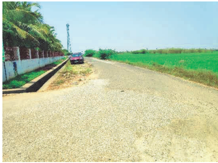
View of access road
