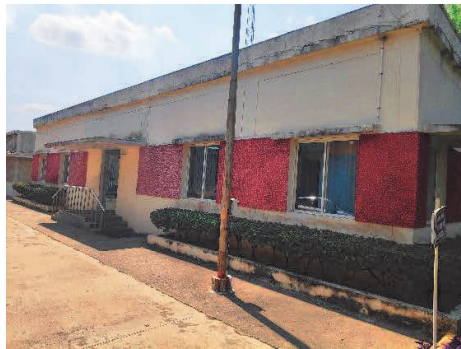
View of the Admin office block
