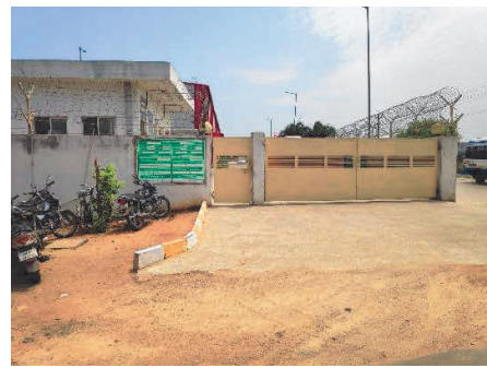
View of Entrance of the property
