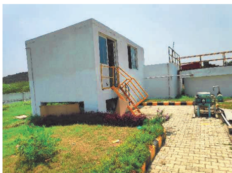
View of the STP room
