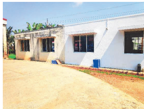
View of the Pump Room
