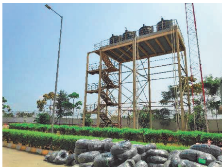
View of the water tank
