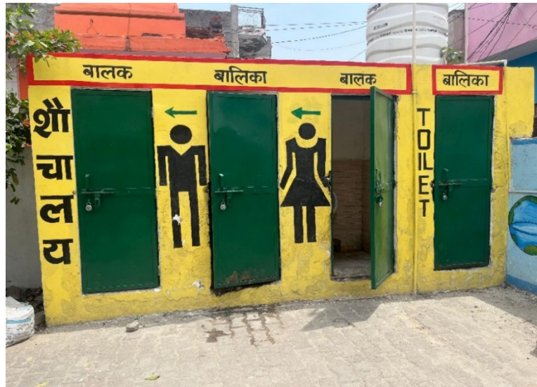
Figure 11: Toilet Facilities, Primary School Dankaur Dehat
