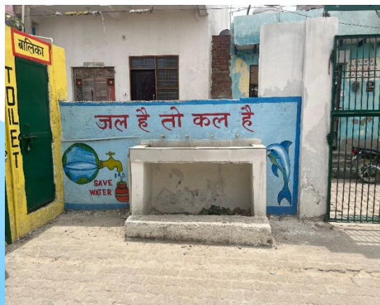
Figure 4: Water taps installed at PS Dankaur Dehat
