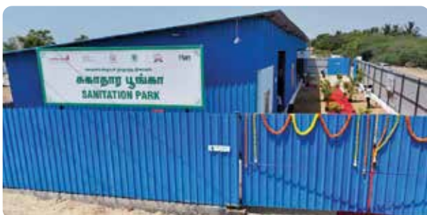
Establishment of sanitation park to segregate and recycle dry waste.
