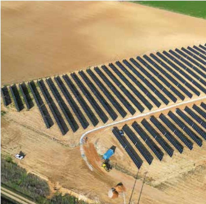
Solar farm in Medina, Spain.
